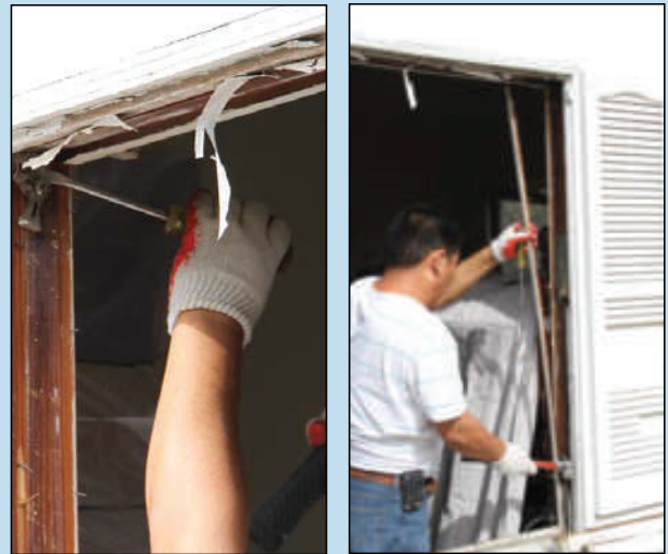
Remove old side trim, nails, and screws
