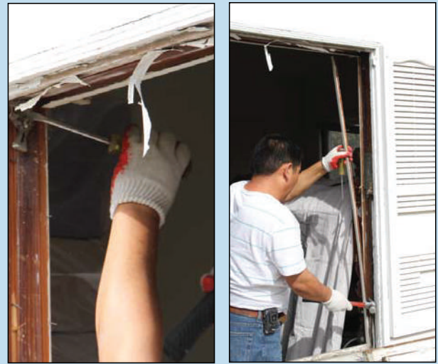
Remove old side trim, nails, and screws
