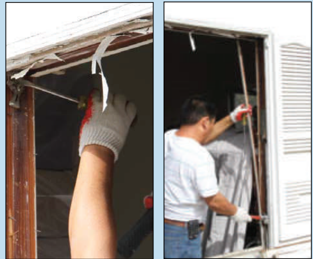
Remove old side trim, nails, and screws
