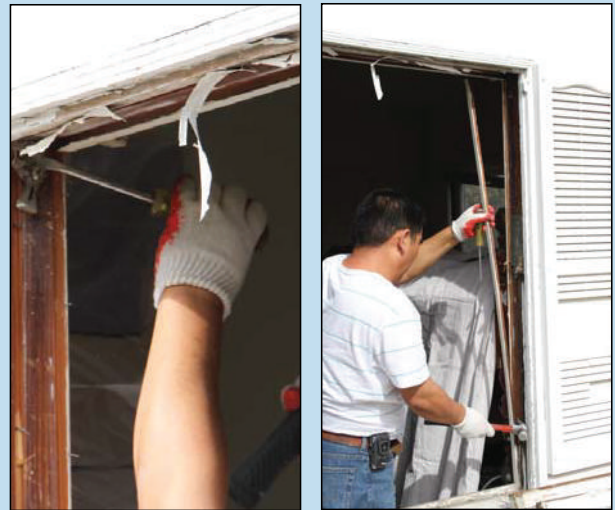
Remove old side trim, nails, and screws
