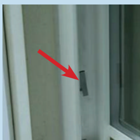
1. Close sash. Flip open balance retaining clip on both sides.
