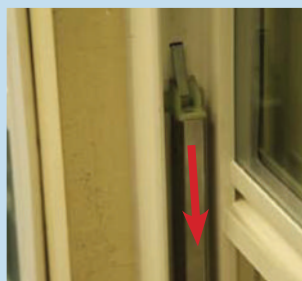
4. Remove balance, lower balance and disengage from balance clip retainer.
