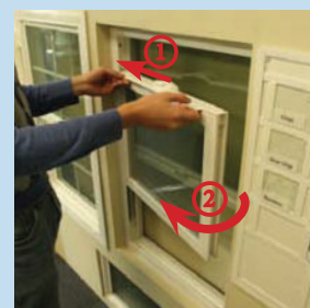
3. Push the sash to one side a little bit. Tilt out sash from one side to remove from frame.
