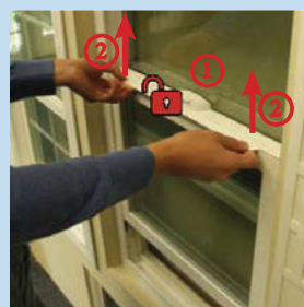
2. Unlock the sash. Then slowly lift sash to fully open position.
