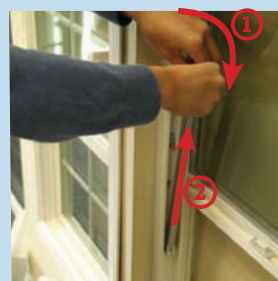
6. Once disengaged remove balance. Tilt out a little. Then lift slowly as balancer will have resistance from the springs.
