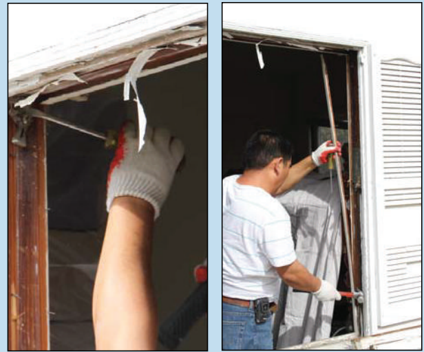
Remove old side trim, nails, and screws
