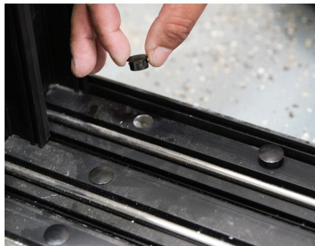
Using silicone press sill hole plugs into place against the jamb.
